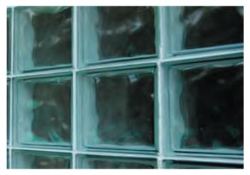
7. **Sista F130 acrylic sealer** was applied as a sealer between all the bricks, and around the outside of the bricks as well.
