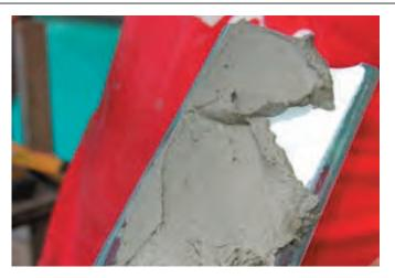
6. Butter the bottom (holding bottom up) and sides of each brick with a liberal amount of mortar mix and lay into position. Repeat until the bottom row is finished. Apply a liberal amount of mortar mix to the top of the first row and repeat this for every following row.
