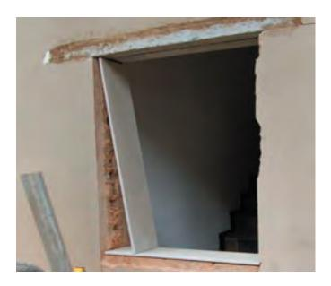
Once the lintel is in position you can safely remove the bricks underneath to open up the space. The bricks need to be cut as cleanly as possible to prevent having to fill in afterwards. Cut 4 fibre cement boards to fit around the opening - you can easily do this with a jigsaw - and screw these into the wall. Using fibre cement board gives a perfect finish to the opening.
