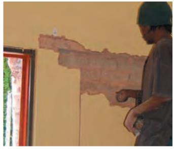
2. Using hammer and chisel the wall was chased out to the shape for the new opening. If you can put up with a ton of dust, you can always use an angle grinder to cut out and a hammer drill to take out the bricks. I did a combination of hand and power tool work to open up the wall. Start at the top and make the opening for the lintel - insert the lintel - **before removing any bricks below this level**.
