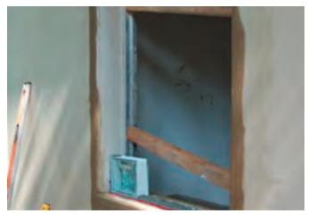
5. Now it's time to start laying the glass bricks. Make sure that the bottom, sides and top are level before you start as you won't be able to fix this later on. For the first course, spread a layer of mortar mix on the bottom of the opening.
