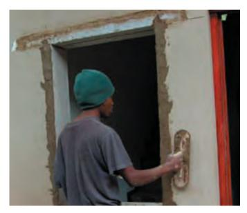
4. Use plaster mix to fill in around the lintel and boards - packing in as much as possible in any openings, and use a float dipped in water to smooth the surface. This will need 2 to 3 days to dry.
